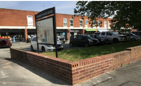
The newly repaired wall at the WP shops
