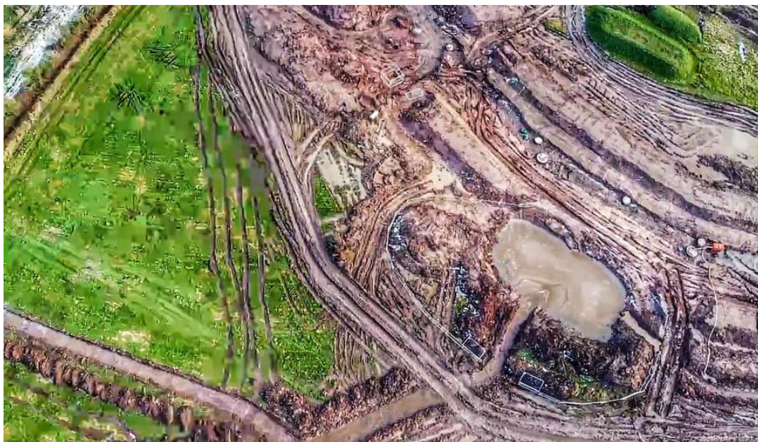
Figure 4: Flooding on Wrexham Road construction site
